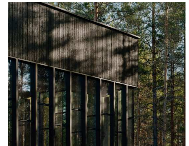
Example of charred, vertical wood cladding and the pattern of shadow cast by the trees.
