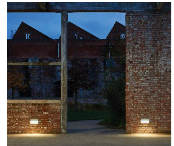
Example of discreet, low-level downlighters.
