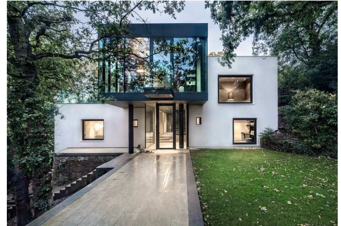
View of the south side showing the house nestled into the trees.
