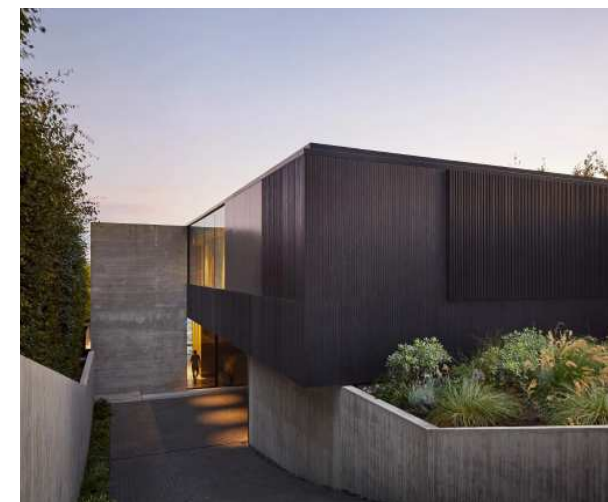
Example of charred, vertical wood cladding combined with a textured concrete, similar to lime render.
