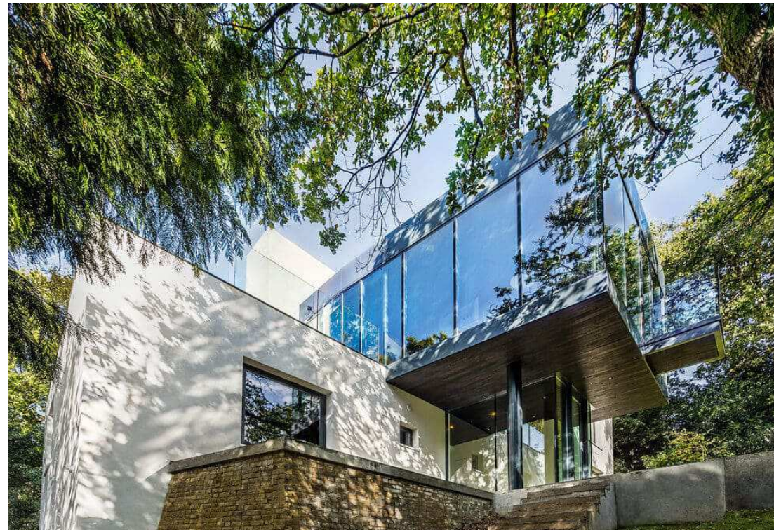
View of the southwest corner.
