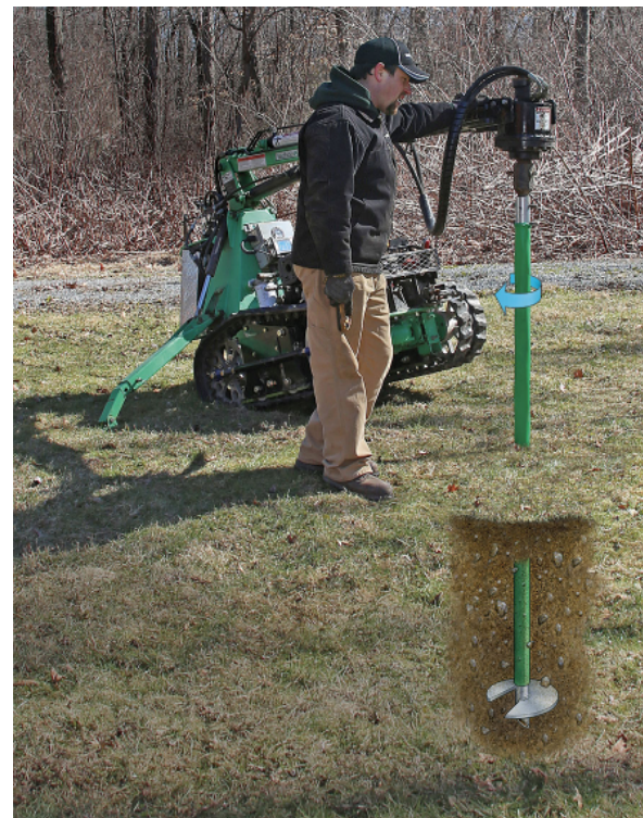
Composite image of a screw-pile being installed.
